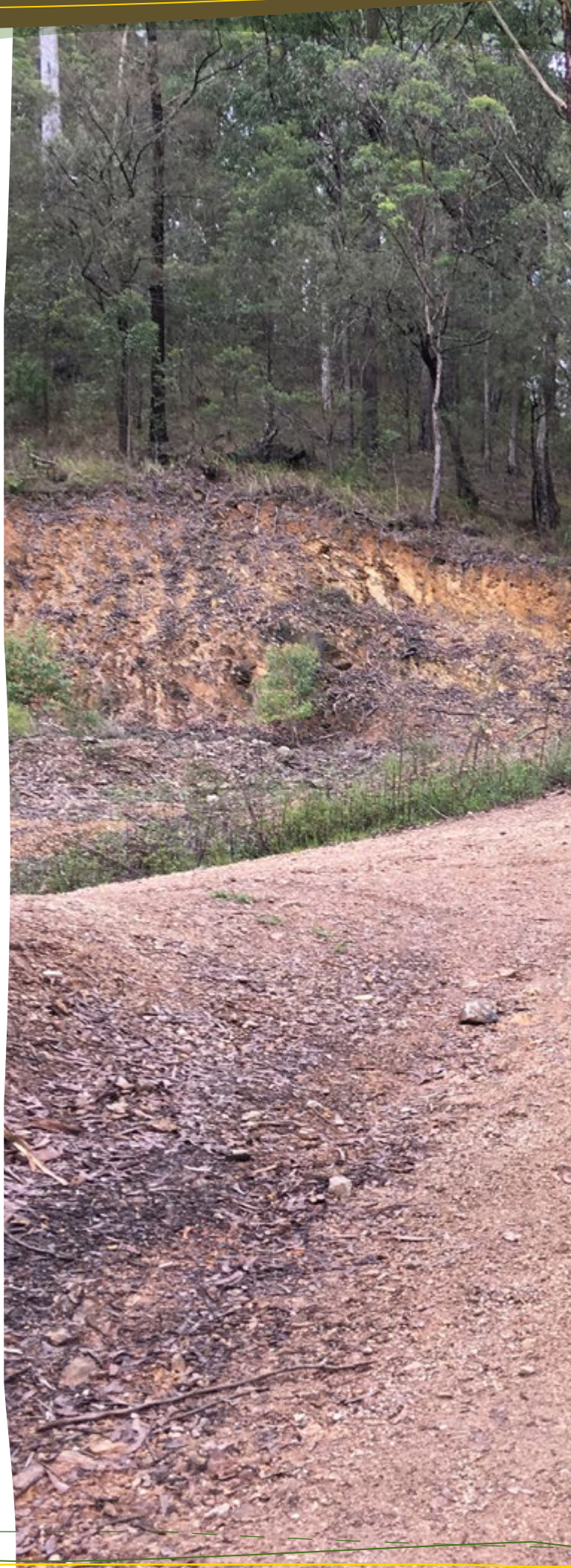
Figure 9: Dispersive sub-soils (score 3) at a road cutting with rill erosion one wet season after grading, with no vegetation growth or colonisation due to the harsh soil environment and erosion.
