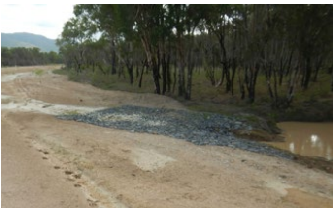
Figure 45: Small rock chutes at diversion drain outlets can prevent gully head-cutting upstream into drains.
