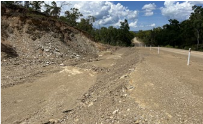
Figure 64: A roadside gravel pit that drains directly to a stream in background via a gully channel outlet.
