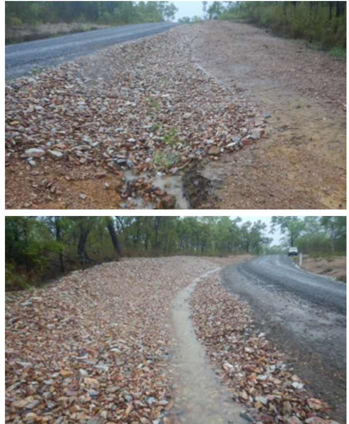
Figure 29: Rock-lined table drains on unsealed roads.
