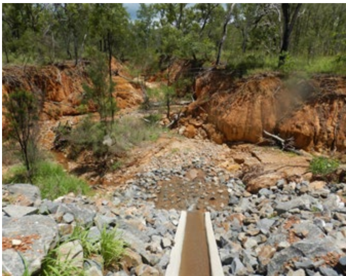
Figure 49: Gully bank collapse downstream of a concrete culvert and concrete chute due to a lack of rock scour protection in the receiving environment beyond the immediate structure (left), and after gully control and rock chute installation (right).
